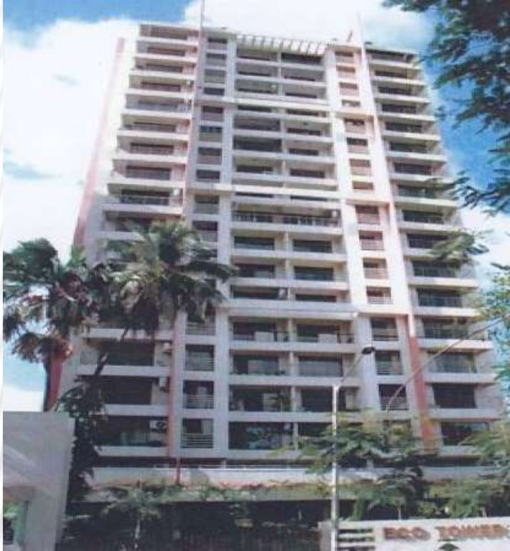
ECO TOWER Andheri ( East ) Eco Homes Constructions Pvt. Ltd.
