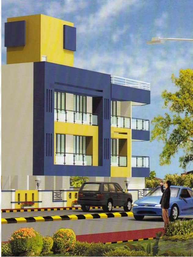
DANI HOUSE Kandivali ( West ) Dani Developer.
