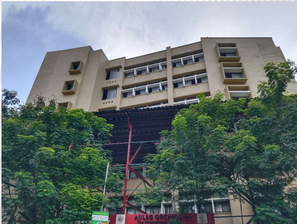
SCHOOL at MULUND (E) Phase 1 completed, Phase 2 Under Construction
